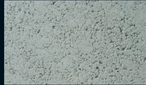
FISSURED AC F02
