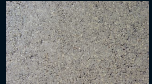
FISSURED AC F06
